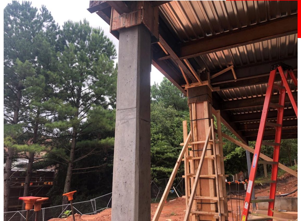
Interior columns formed and poured
