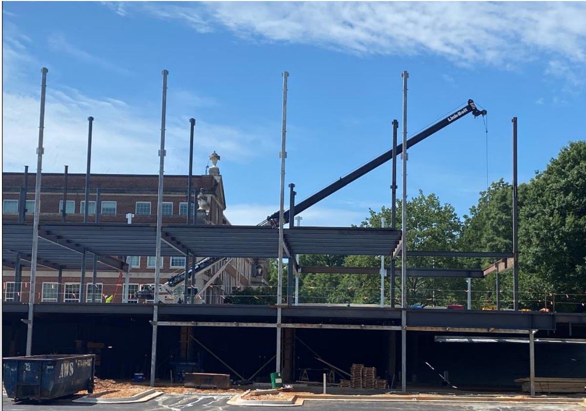
Steel erection at new addition
