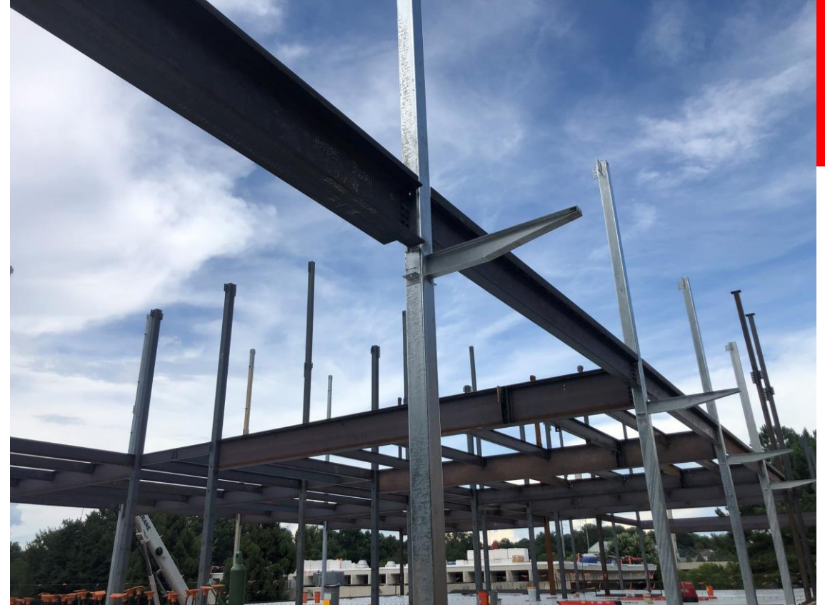
Third floor perimeter steel installed at new addition
