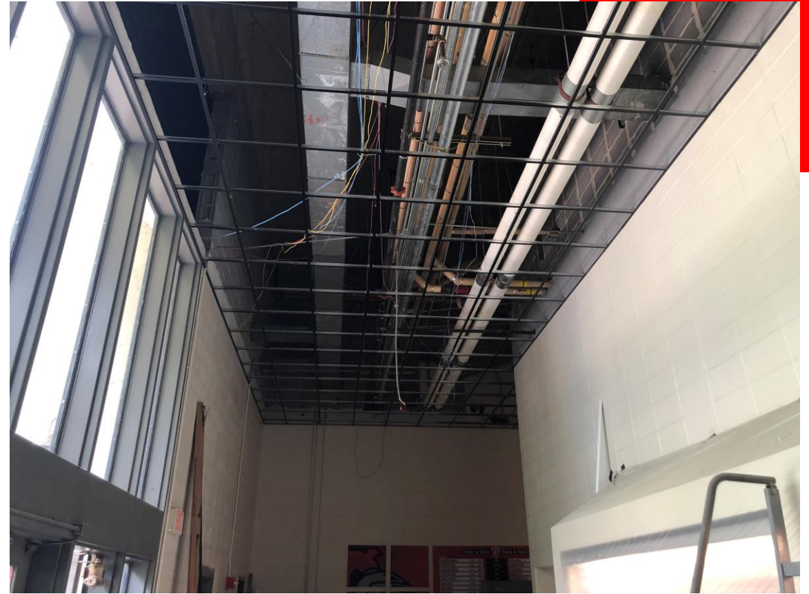
New Ceiling Grid installed in Performance Gym Lobby
